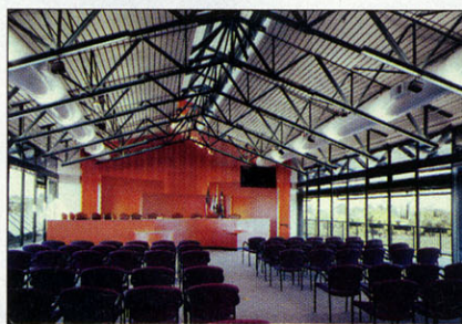
The third-floor council chamber with gable manufactured joists and continuous window walls.
