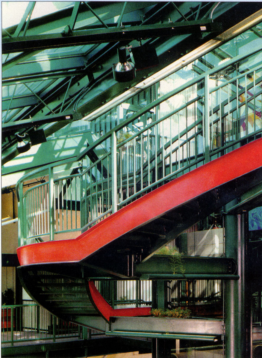
Steel "branches" extend from the central pipe (or trunk) to support the stairs.
