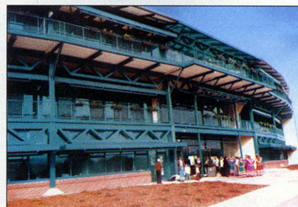
The Civic Center on opening day. The top chords of joists extend to create cantilevered exterior decks.
